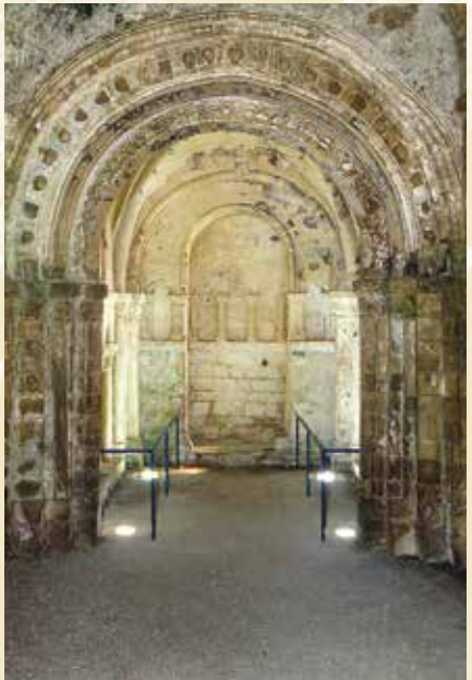
Interior of Cormac's Chapel
